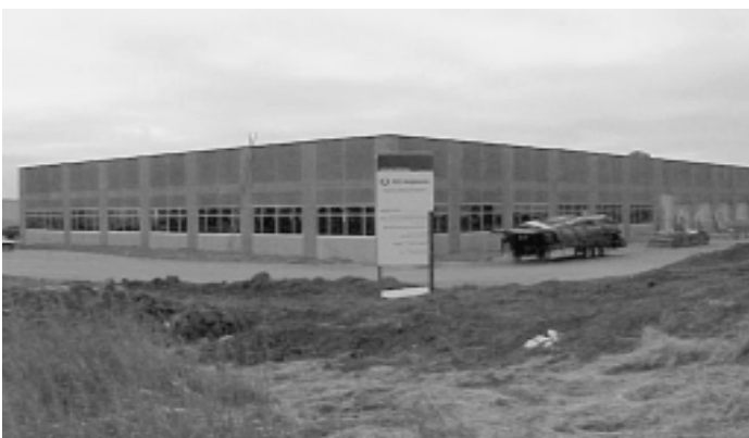
Ground breaking for JDSU, Fall 2002
